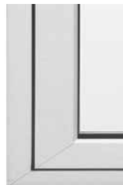
Outside: window sits flush within the frame.
