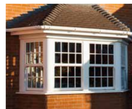
Bay window with vertical sliding sash windows
